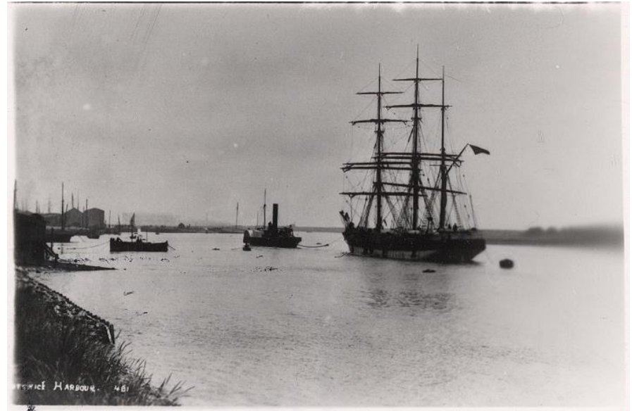
Figure 17. Shoreham harbour, 19 th century
